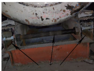
图2 基础加强 Fig.2 Strengthened foundation
